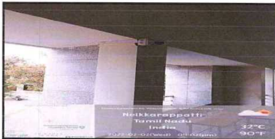
CCTV- Admin Block First Floor
